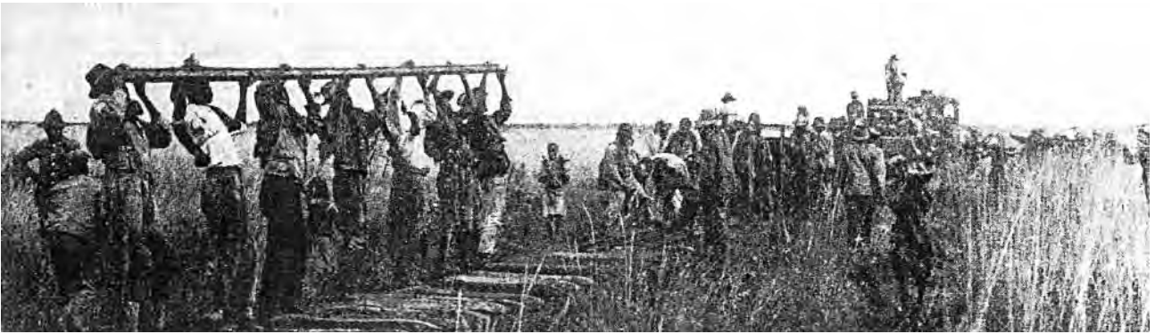
Construction of the Otavi Railway.
